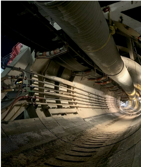
TBC “Vegas Loop” tunneling project
