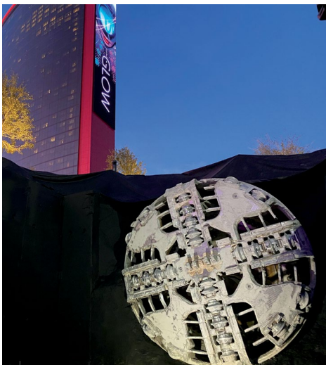
TBC “Vegas Loop” tunneling project
