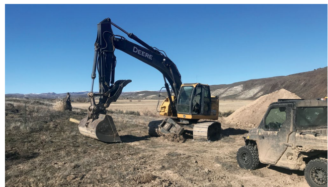
The John Deere 225DLC excavator and the UTV
