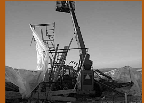
A Grand Traverse Construction employee was struck and killed by this scaffolding that overturned due to high winds.
