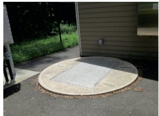
Permit required confined space danger sign not posted at a water pollution control facility wet well entrance.
