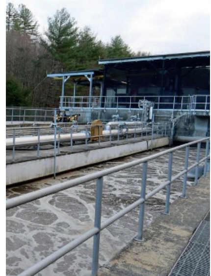
Rails at the water pollution control facility are not compliant with fall protection requirements.
