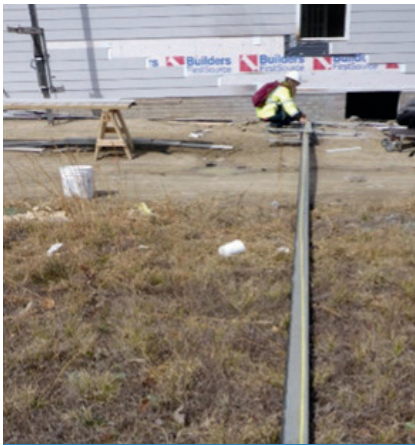
Depiction of the VOSH Compliance Safety and Health Officer taking measurements of the pole that contacted the overhead powerline.
