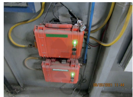
Grade D breathing air system for the supplied air respirator.
