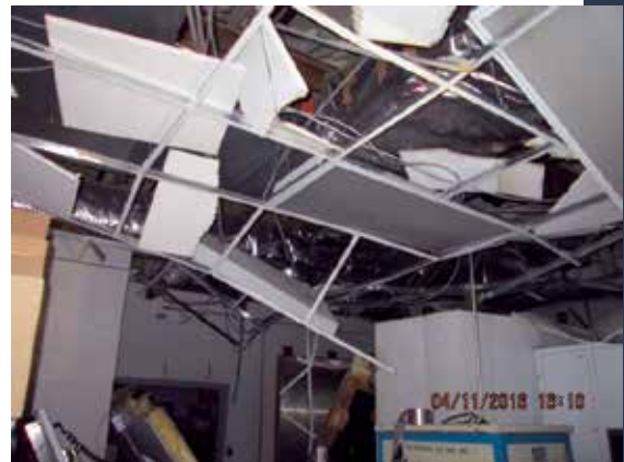
Research chamber local exhaust system ductwork exploded in the ceiling.
