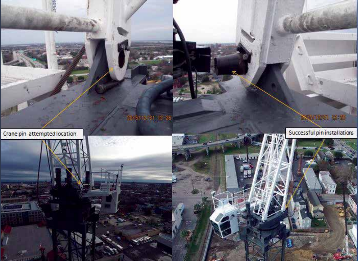
Crane pin attempted and successful pin installation on tower crane
