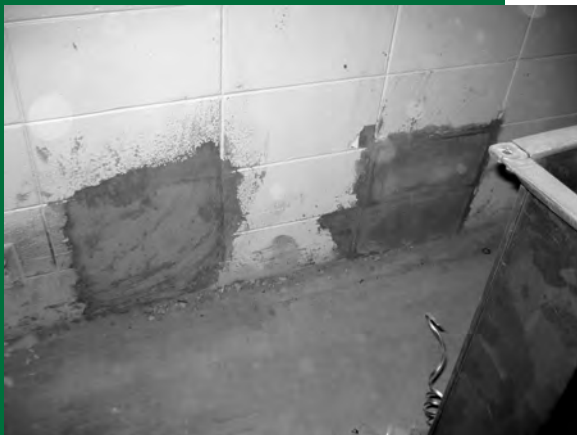
Wall holes containing ACM
