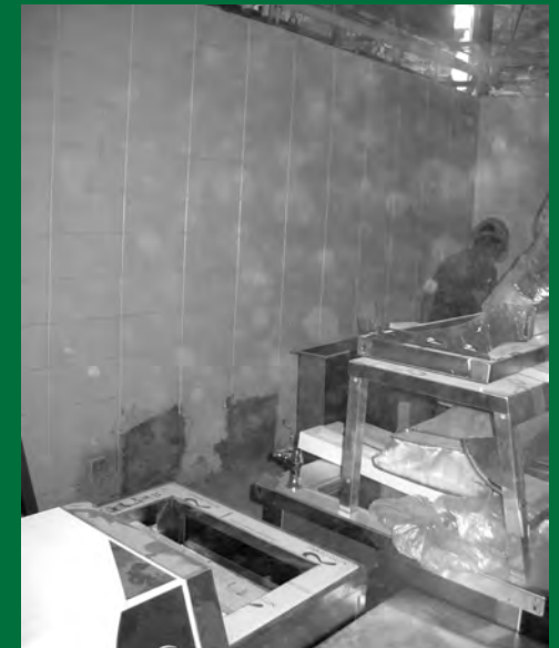
Area filled with asbestos dust
