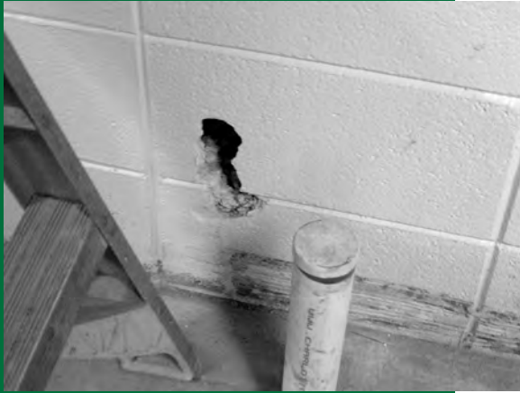
Wall hole for drain line
