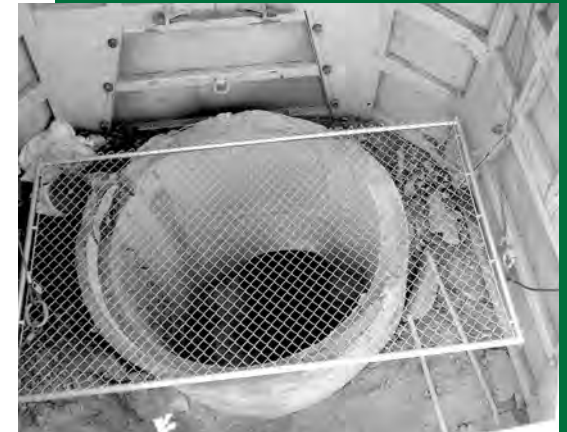
A worker was overcome by carbon monoxide while using a gas powered saw in this manhole.
